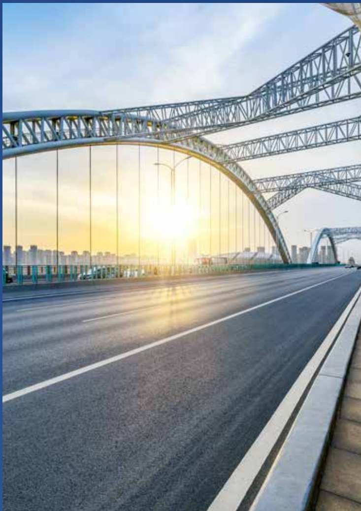
Kopri Bridge Widening
