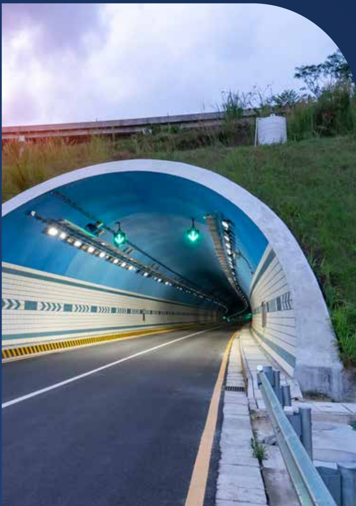
Thane - Borivali Underground Tunnel
