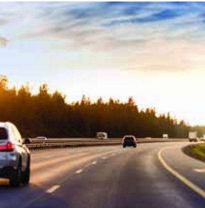
CENTRAL PARK ROAD LINKING KOLSHET & BHIWANDI
