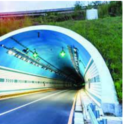
BORIVALI - THANE TUNNEL
