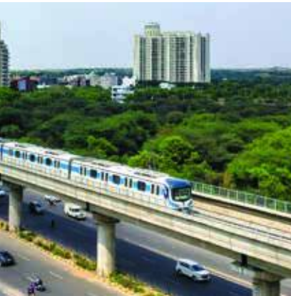
MUMBAI METRO LINE 5
